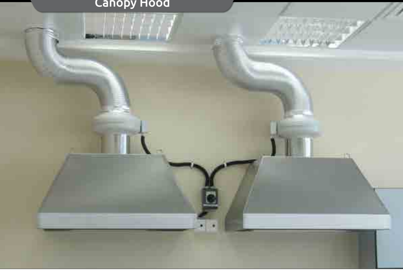
Ceiling mounted and wall mounted canopy hoods.
